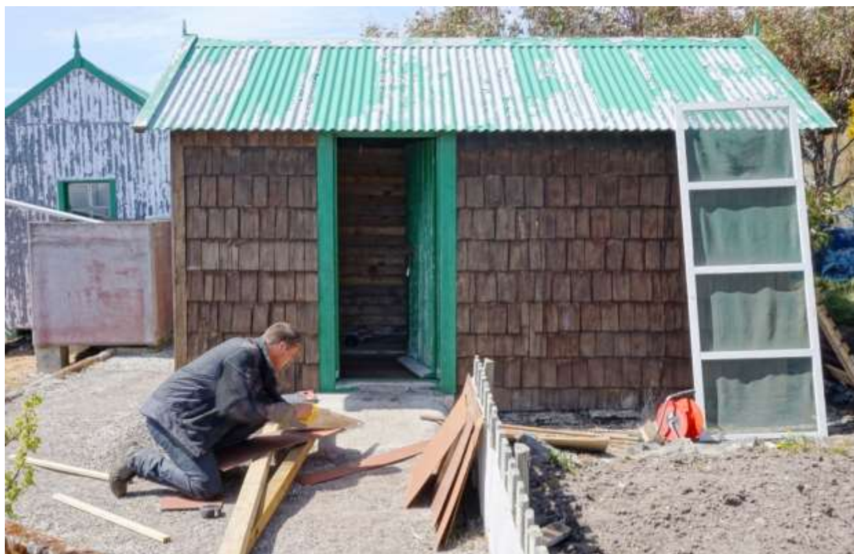
Figure 1: Refitting a shed into a makeshift quarantine facility.
